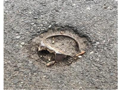
**GAS TURN-OFF VALVE CAPS.** You can also monitor the condition of gas turn-off valve caps. Look for the gas turn-off valve caps on your street. When a gas turn-off valve is paved over or if the cover is in bad condition, it can be hard to turn off the gas in case of a fire.
